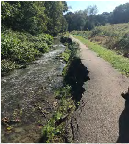
Erosion is degrading former golf cart paths, which were constructed too close to Chalfant Run
