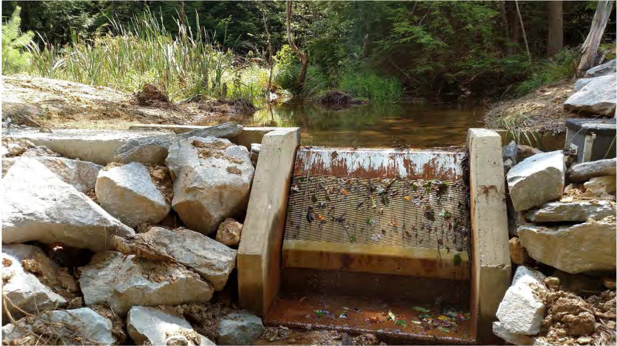
Photo 1. A stream intake structure that collects and diverts a maximum flow of water to a treatment facility while bypassing flow above the maximum. The screen prevents debris from plugging the transfer pipe
