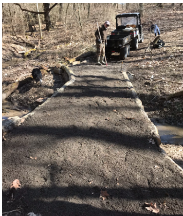
A “during” and “after” of Audubon Greenway’s stream crossing. On the left, a pipe is being installed to continue water flow. On the right, is the finished bridge, connecting trails on either side of the stream. Photos by April Claus.
