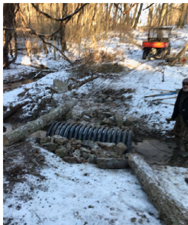
A “during” and “after” of Audubon Greenway’s stream crossing. On the left, a pipe is being installed to continue water flow. On the right, is the finished bridge, connecting trails on either side of the stream. Photos by April Claus.
