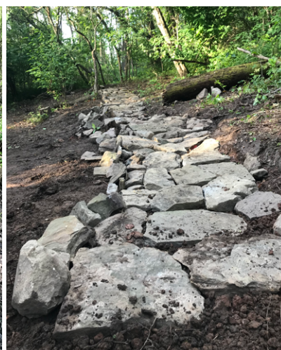
A “before” and “after” of Dead Man’s Hollow’s Cool Spirit Trail. On the left, water damage is apparent, and on the right is the rock armoring used to address the issue. Photos by Caitlin Seiler.
