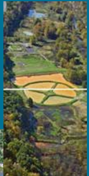
Wingfield Pines AMD treatment system
