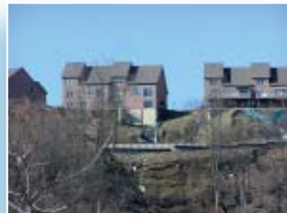
Tree removal and grading too close to the ridgeline caused a serious landslide exposing building foundations. Walls are being built in an attempt to stabilize the site, and black plastic being used to prevent water from further saturating the soils. This landslide scar will take decades to heal.
