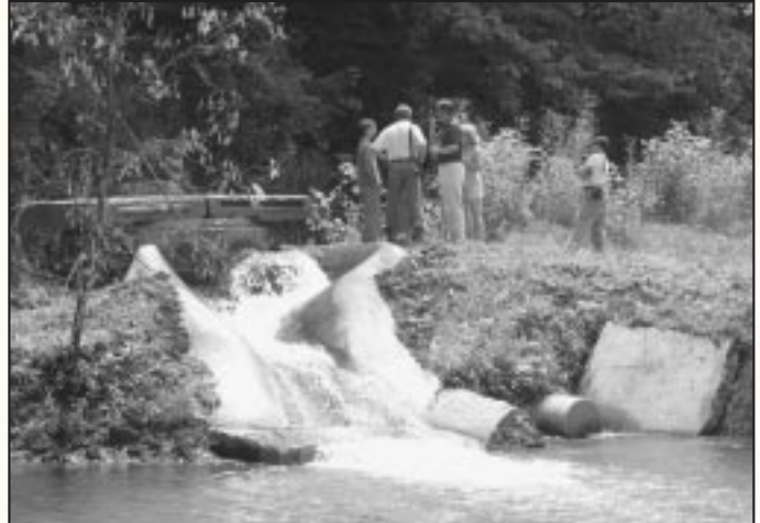
The 2000-gallon-per-minute iron laden discharge at Wingfield Pines is being plumbed to raise its elevation so the water can circulate through a settling system.
